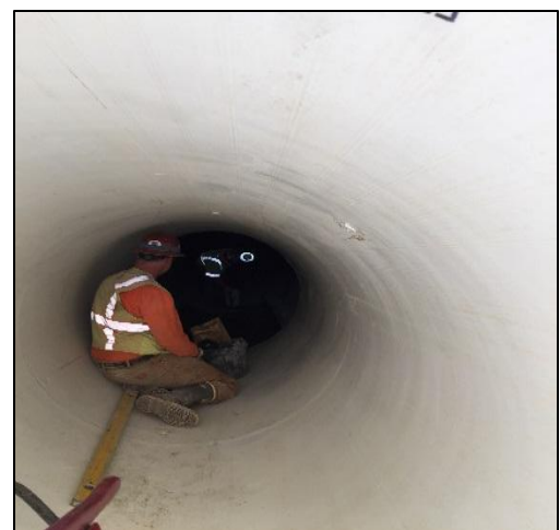
RCP T-Weld Inspection
