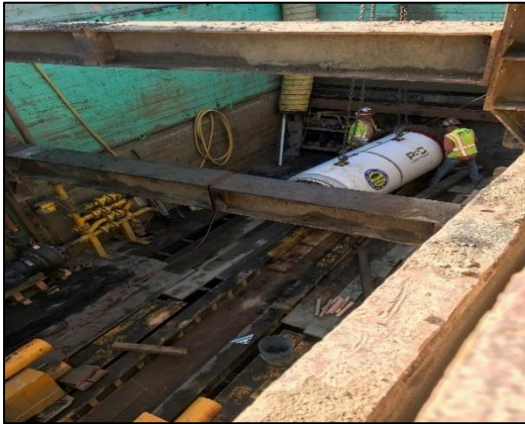
Micro-tunneling carrier pipe installation
